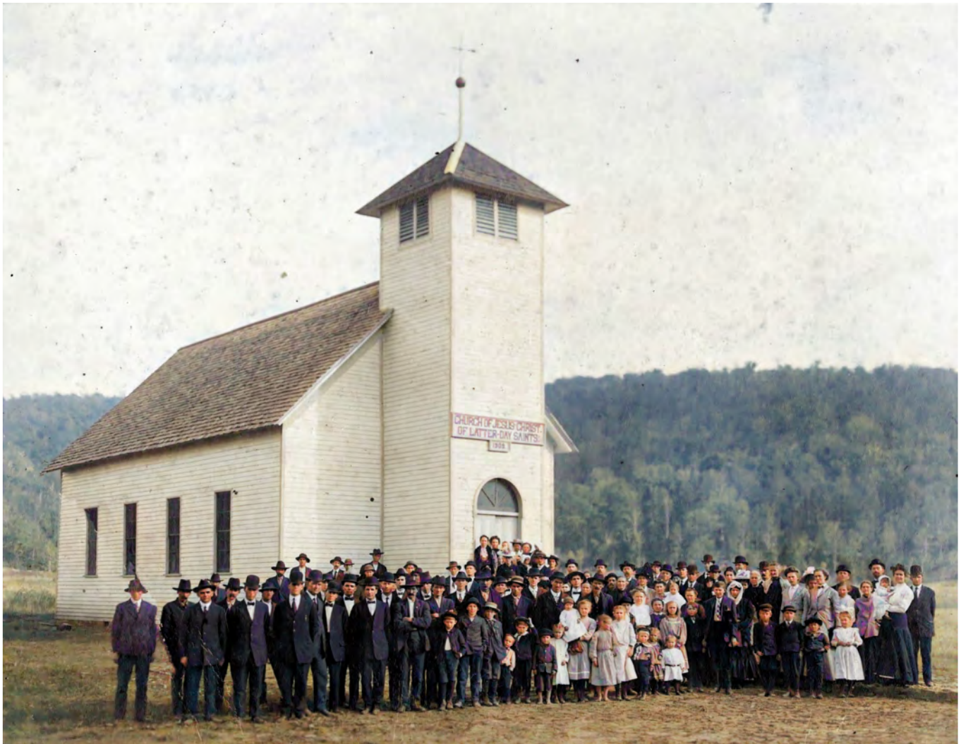
Northcutts Cove Chapel Dedication October 24, 1909
